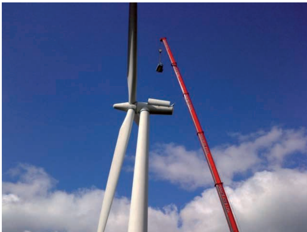
A generator exchange in progress
