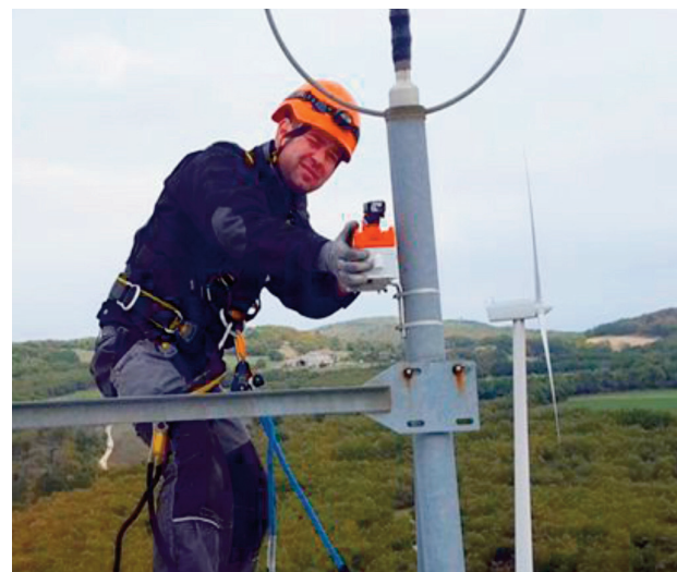
Rotor balance diagnostics and sensor alignment on a TRIG site in France
