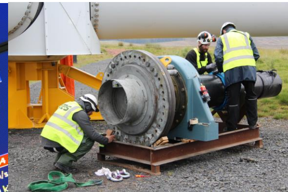
Main bearing replacement underway
