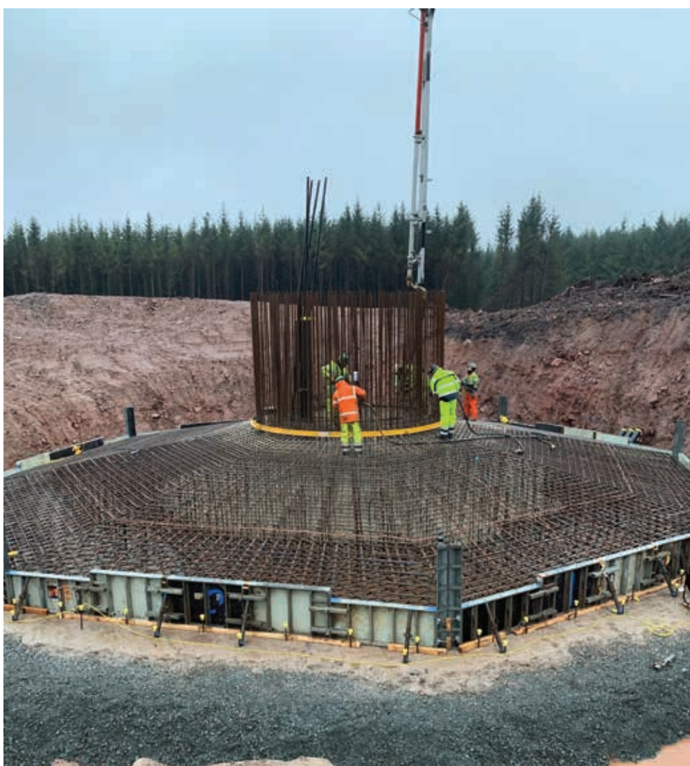
Local Contractor, Hansons, pouring concrete for a foundation at Solwaybank Wind Farm, December 2018.
