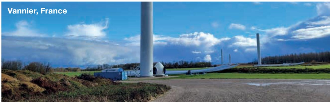
Located in the Haute-Marne department in France, Vannier is a 43MW onshore wind farm consisting of 17 Envision E-131 2.5MW turbines. Construction commenced in February 2020, with TRIG acquiring Vannier in October 2020. Construction is being delivered under an EPC wrap by an Envision-Velocita consortium, with RES hired as Owner's Engineer to provide independent construction monitoring.
